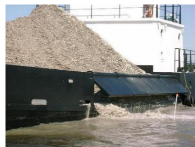
Figure F.7: Depositing Oyster Shell, Raritan Bay, USA Source: Baykeeper webpage, New Jersey
