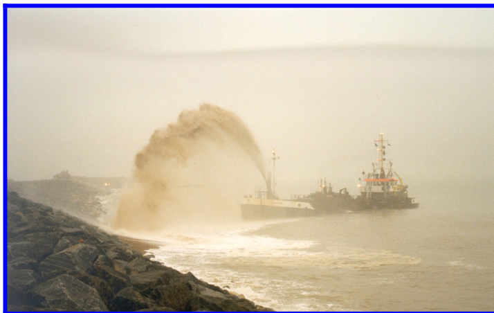
Figure 5.3: Foreshore Sediment Recharge.
