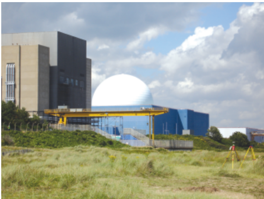
1.64 million tonnes of marine aggregate were used in the construction of Sizewell B
