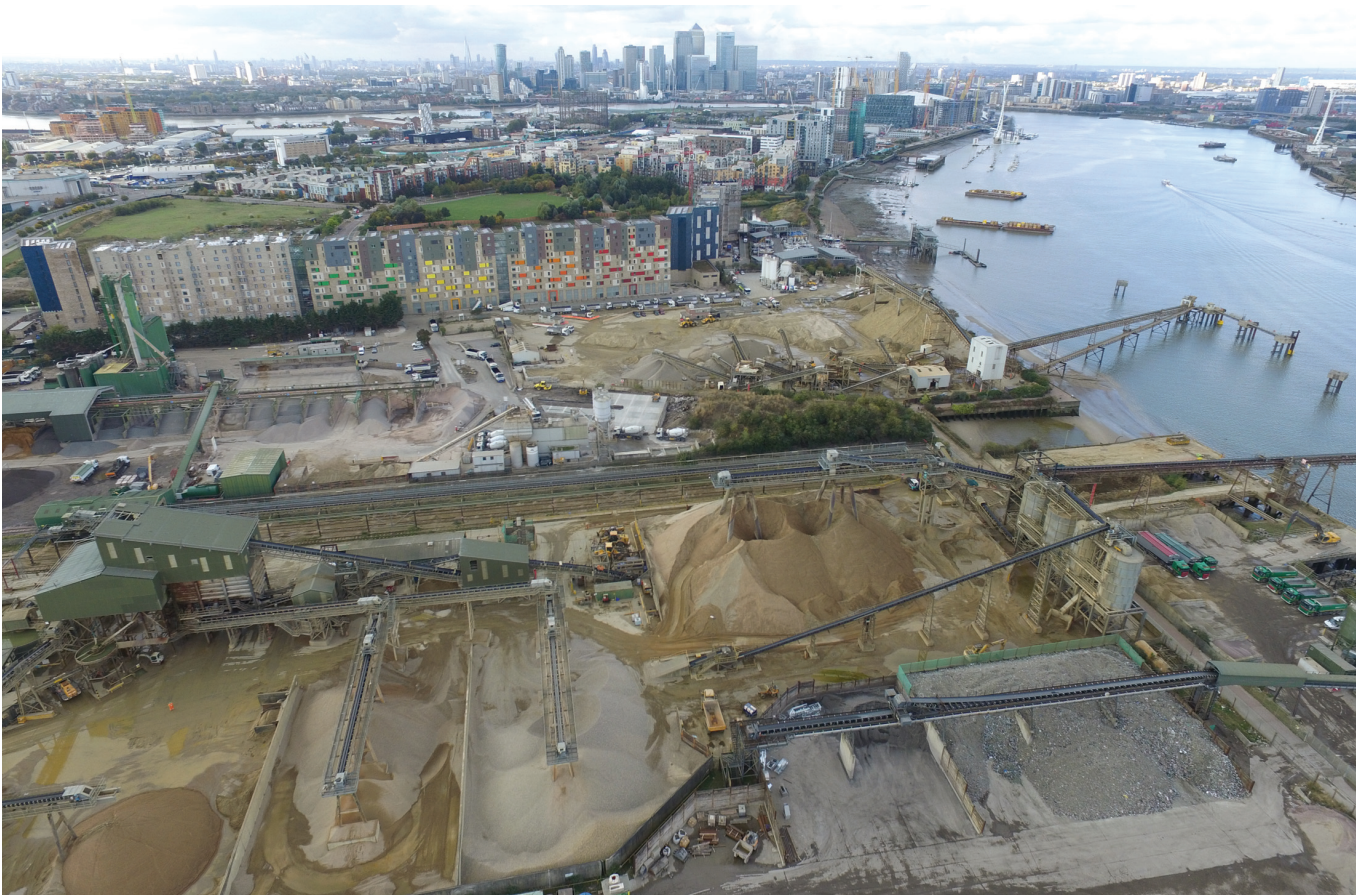
Figure 3. Aerial photograph of Tarmac Marine's dedicated marine aggregate wharf and processing plant at Greenwich on the River Thames, looking west towards central London. Note the plant's rail freight loading facility and the close proximity to the site of the newly constructed residential flats in the foreground.
